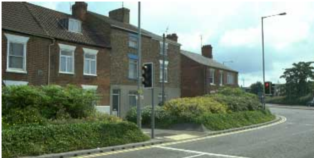
Raised beds These planters have no highway function, and are thus coded as EFC/LE7.2
