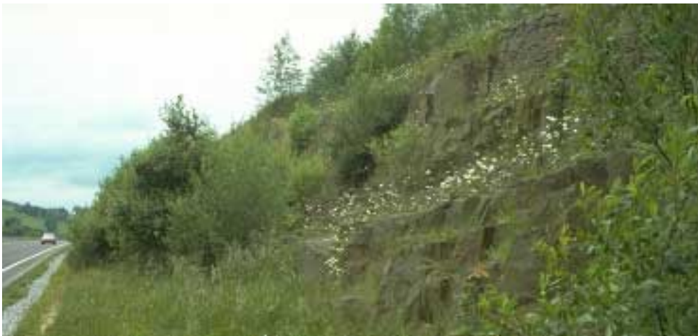
Scrub and Tree Seedlings Control of volunteer tree seedlings and scrub may be necessary to prevent encroachment over ground flora, and for safety reasons
