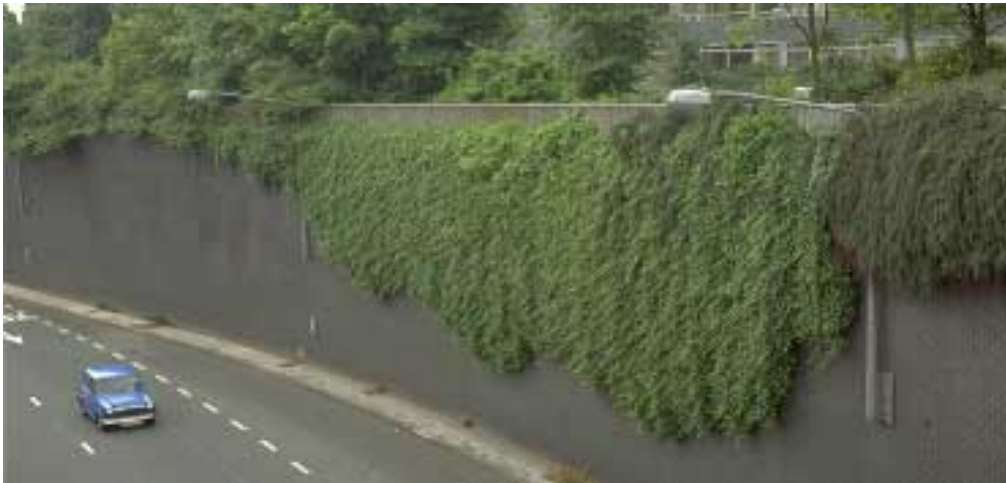
Trailers Structures and boundaries can be softened by trailers but access and maintenance problems need to be resolved at the design stage
