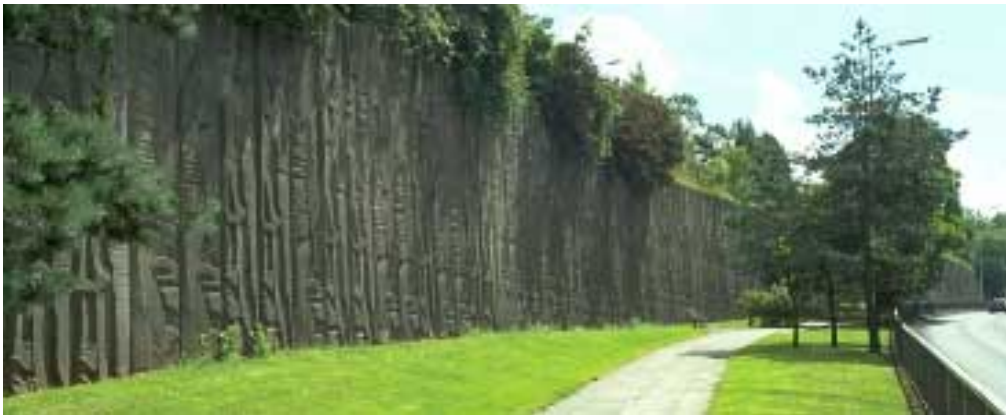
A451 Retaining Wall Relief Structural finishes can provide a dramatic feature and are set off by amenity grass within the public open space nearby
