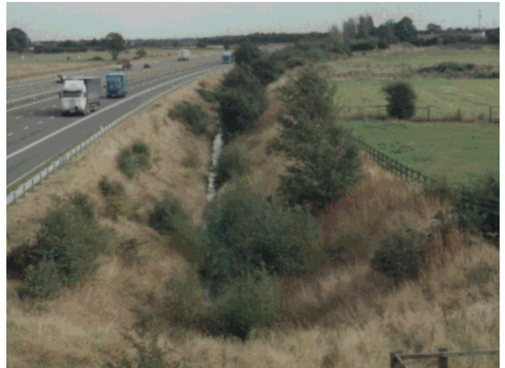
M62 Humberside Drainage Channels Open ditches for agricultural drainage within motorway boundary
