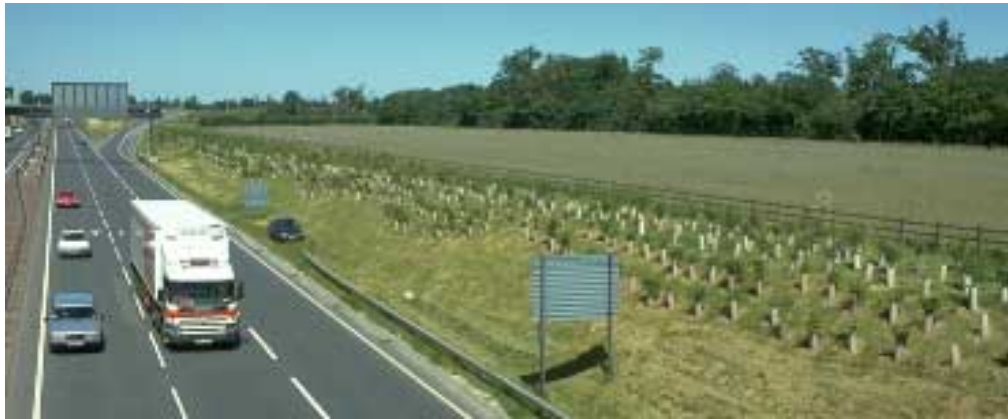
A11 Tube Forest This linear planting is not required for Screening, and also prevents Landscape Integration by imposing an artificial barrier and highlighting the highway boundary
