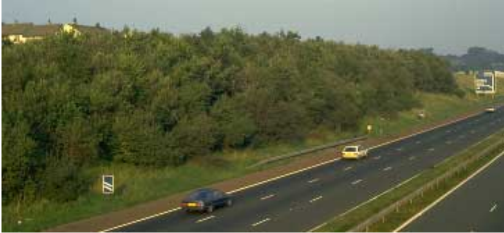
Planted Screen Planting to provide Screening for residential property. It has also been extended down to the cutting to better integrate the earthworks into the landscape, and provide interest to road users; Secondary Function EFB
