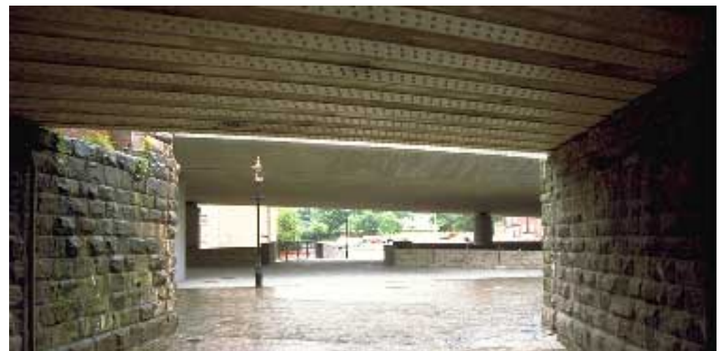
Bridge Underside Bats may roost under bridge decks and these should be inspected prior to maintenance operations
