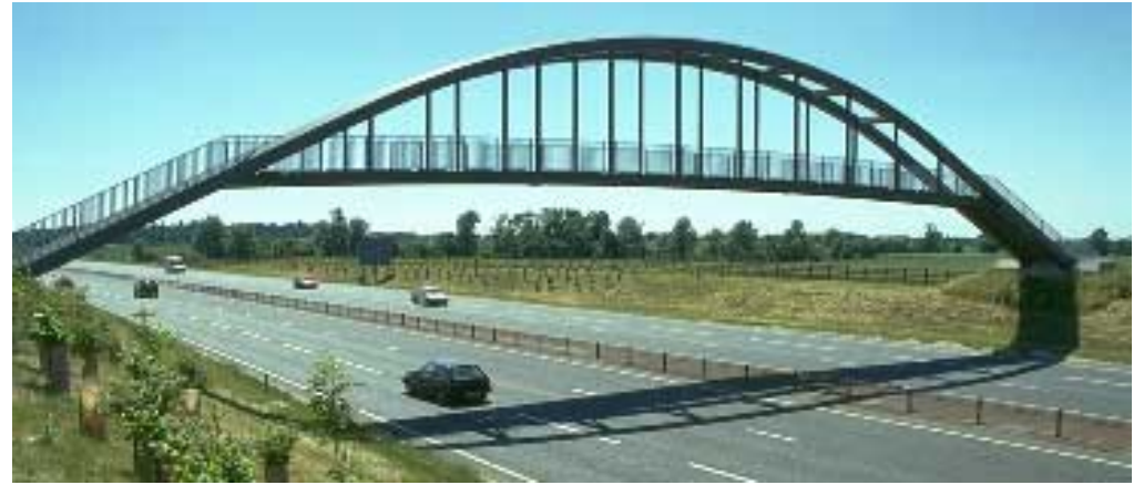
A11 Footbridge Detailing the shape and finishes on the majority of structures, emphasises their dramatic effect, and can enhance the sense of arrival
