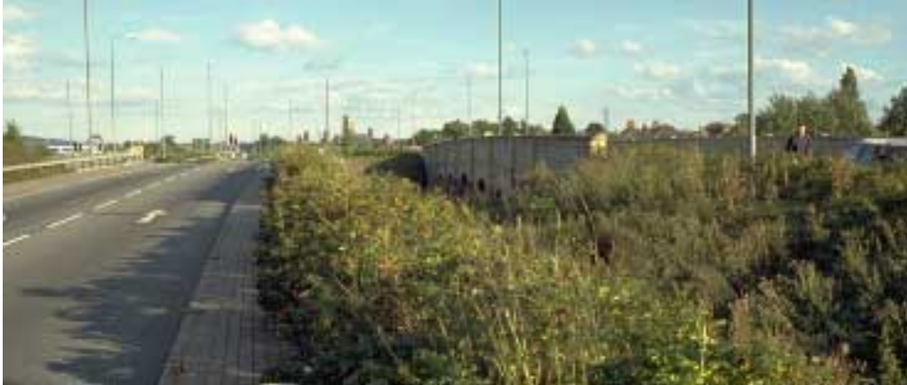
Ornamental hedge Ornamental hedge provides a formal treatment with structural planting benefits
