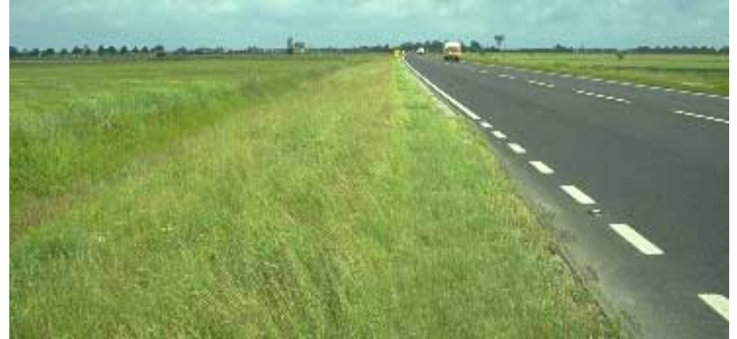
A17 Flat Landscape The absence of boundary fences retains the road's relationship with the traditional landscape
