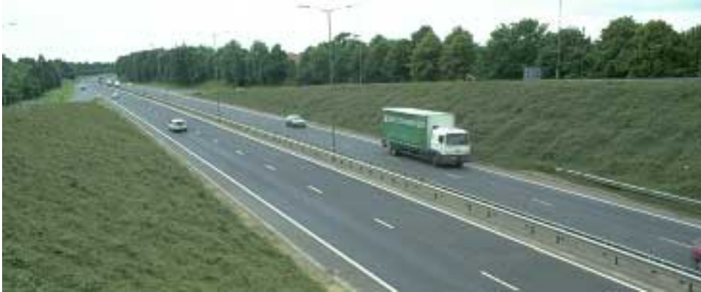
Groundcover Formal treatments to urban interchanges
