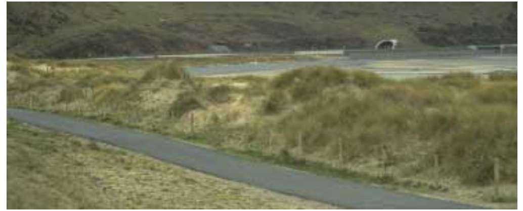
A55 Dunes Specialist soil and vegetation restoration techniques may be specified to achieve a seamless interface with adjacent land and mask the highway boundary. Such areas will need ongoing management to achieve their objectives
