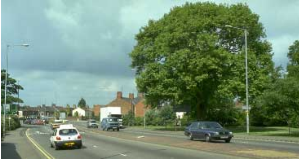
Plane retained Retained during construction
