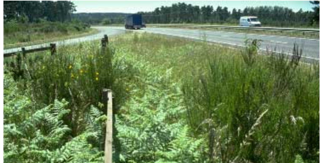
Thetford Heath Locally indigenous flora encouraged into verges from adjacent heath by limiting routine maintenance
