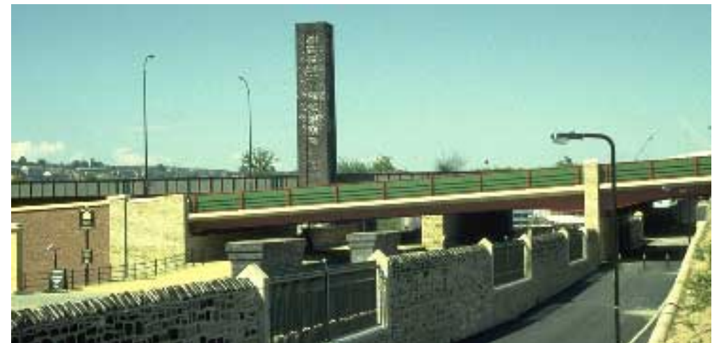
Victoria Quays Hard landscape and urban design skills blend the historic and modern features
