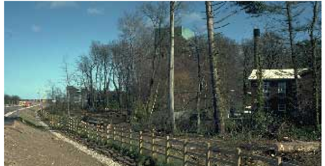
Tree roots/safety barriers Even minor highway works can damage tree roots unless properly supervised with prior specialist input
